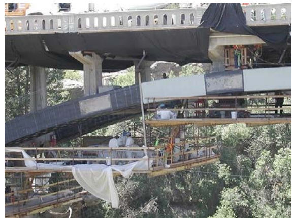
Fig. 12. Strengthening of a concrete bridge with the CFRP sheets, [15].
