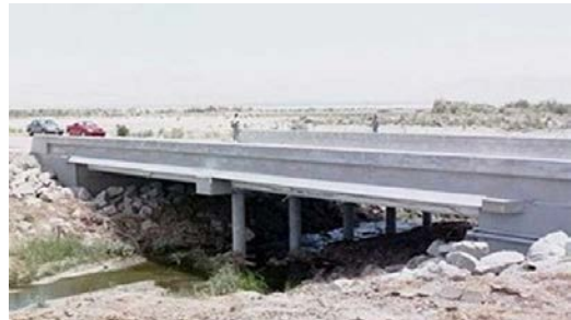
Fig. 3. King's Stormwater Channel Bridge, [8].
