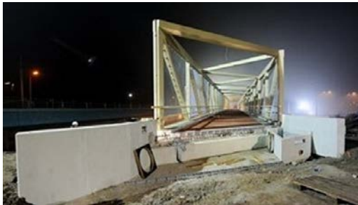
Fig. 2. Hybrid bridge over A27 motorway near Utrecht, [7].
