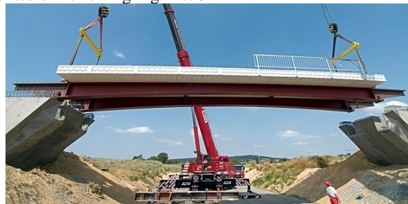
Fig. 5. Friedberg bridge over B3 highway, [10].
