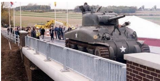
Fig. 6. West Mill bridge (Oxfordshire, 2002), [11].
