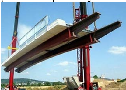
Fig. 4. Friedberg bridge over B3 highway, [9].
