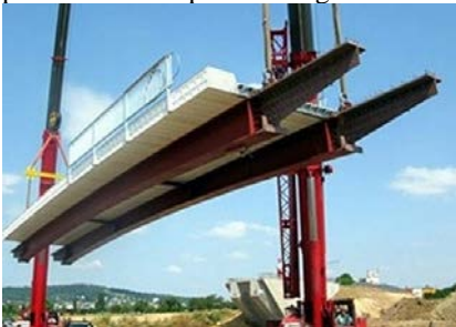
Fig. 4. Friedberg bridge over B3 highway, [9].
