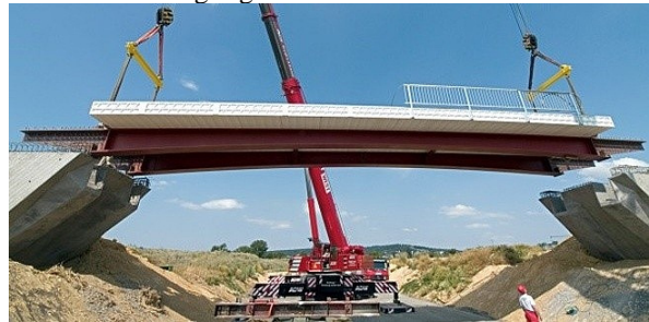
Fig. 5. Friedberg bridge over B3 highway, [10].
