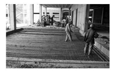
Figure 1.10 GFRP reinforced-concrete slab (Oran, Algeria).
