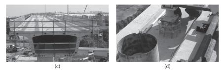
Figure 1.11 GFRP reinforced-concrete rail track structure: bars in concrete rail plinths ((a) and (b)), deck bars for segmental precast elements (c), and high voltage pedestals in overhead rail guideway (d) (Miami, Florida).
