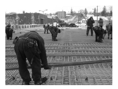
Figure 1.6 GFRP reinforced-concrete bridge deck (Cookshire-Eaton, Quebec, Canada).
