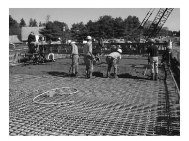
Figure 1.5 GFRP reinforced-concrete bridge deck (Morristown, Vermont).
