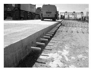
Figure 1.3 Dowel bars in concrete pavements (Port of Rotterdam, The Netherlands).
