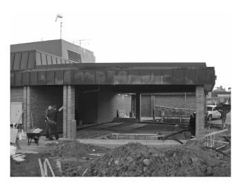
Figure 1.9 GFRP reinforced-concrete slab for MRI rooms in hospital (York, Maine).
