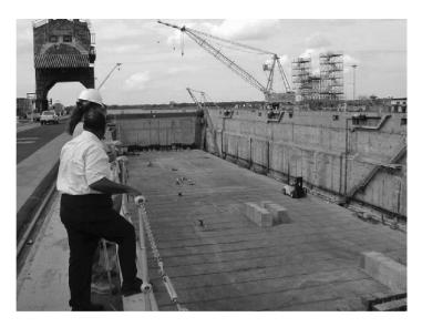
Figure 1.4 GFRP reinforced-concrete repair for Pearl Harbor dry docks (Honolulu, Hawaii).
