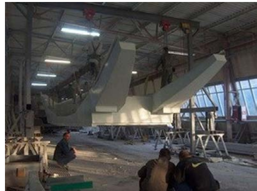
Fig. 9. ApATeCh arched footbridge (Produced by vacuum infusion), [12].
