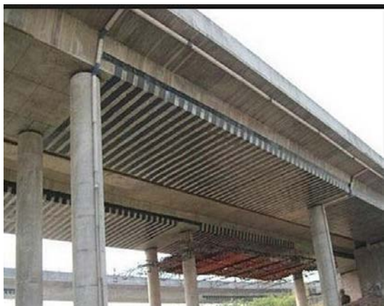
Fig. 11. Strengthening of a concrete bridge with CFRP strips, [14].
