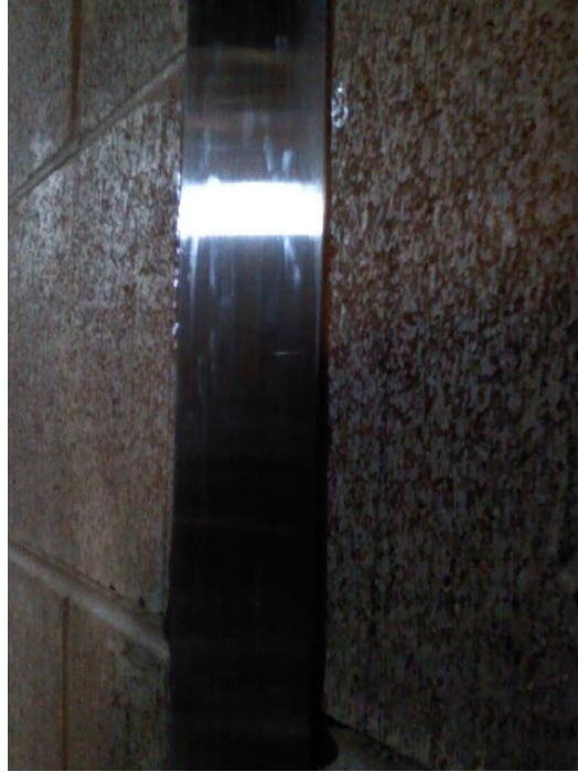
Figure 11 CFRP Plate bonded to a masonry wall
