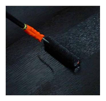
Belzona 5813 is a solvent-free, two-component static dissipative barrier coating.
