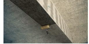
Applying epoxy resin adhesive
