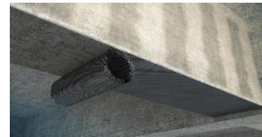
Pasting carbon fiber cloth
