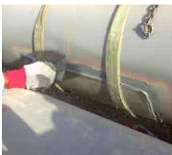
Bonding and shimming
