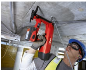
Threaded rod attachments to concrete
