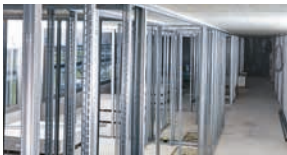
Drywall tracks to concrete and steel
