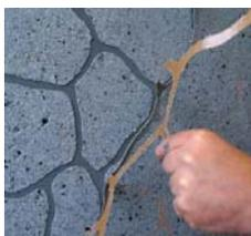
Decorative template than can be used to create brick and stone pattern on facades and walls. The product should be used together with Tytan plasters.
