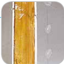
Interior & Exterior Wall Sealing
