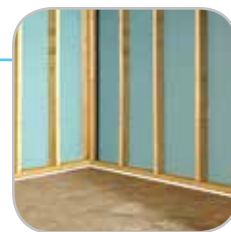
Sill Plate Sealing
