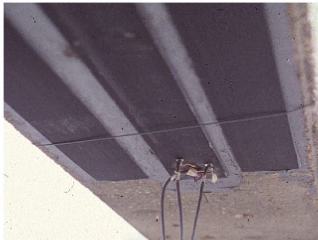
Figure 10 CFRP Plates bonded with epoxy to a concrete beam
