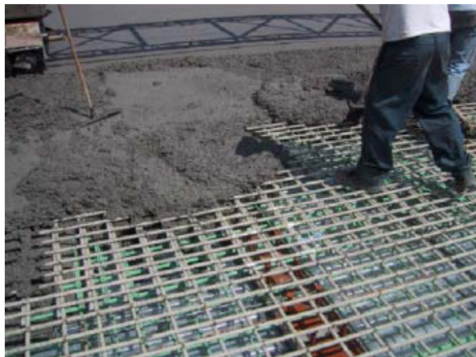
Placing concrete in a bridge slab reinforced with glass FRP bars (top layer) and epoxy coated steel bars (bottom layer)
