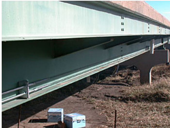
Photo of the Strengthening of Steel Girder Bridge Using Post-tensioned FRP Rods/Strands
